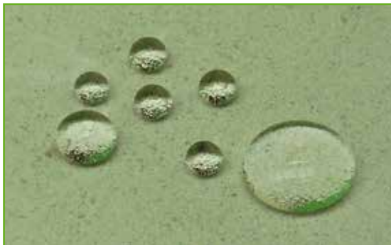
Hydrophobing : Making the building material water repellent
