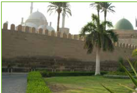
Example for rising damp
