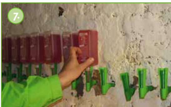
7. The KÖSTER Crisin® 76 cartridges are installed.
